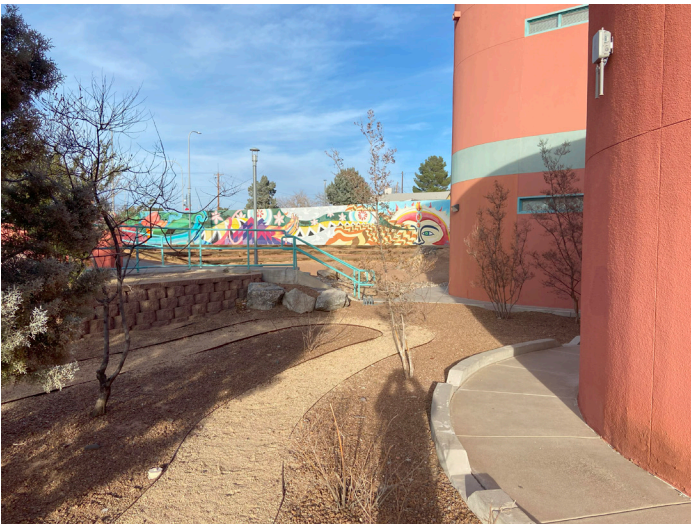
EXISTING RECESSED LANDSCAPE AREA - NORTH SIDE
