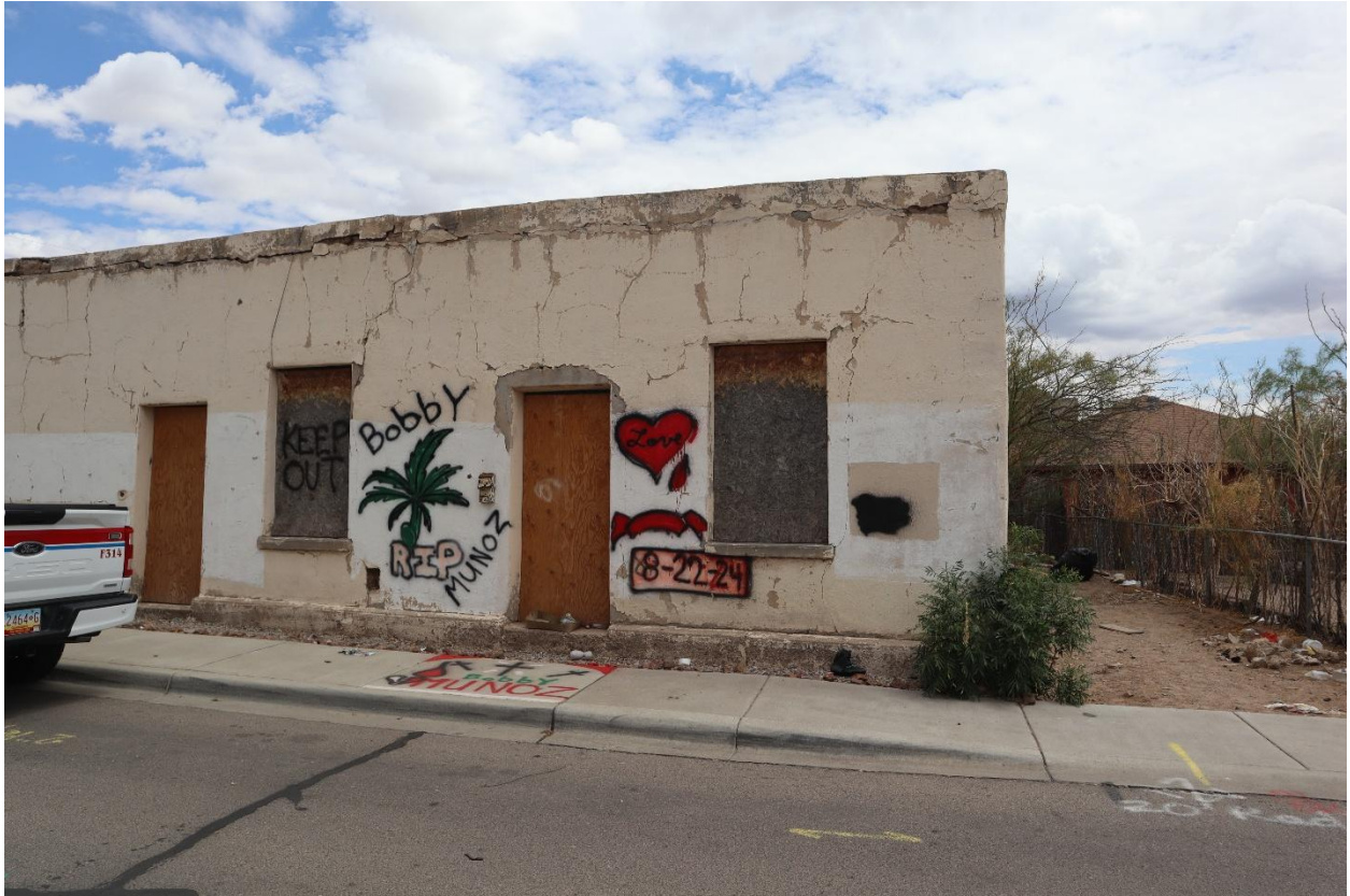
Figure 1: Front façade of 414 E. May Avenue. Photo taken July 1, 2025.
