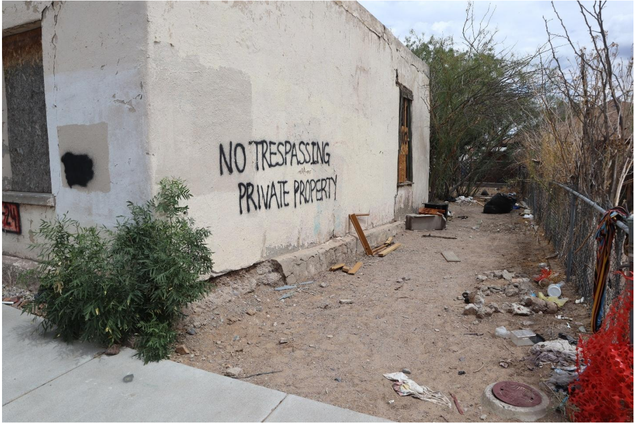
Figure 4: Side access to rear of property at 414 E. May. Photo taken July 1, 2025.
