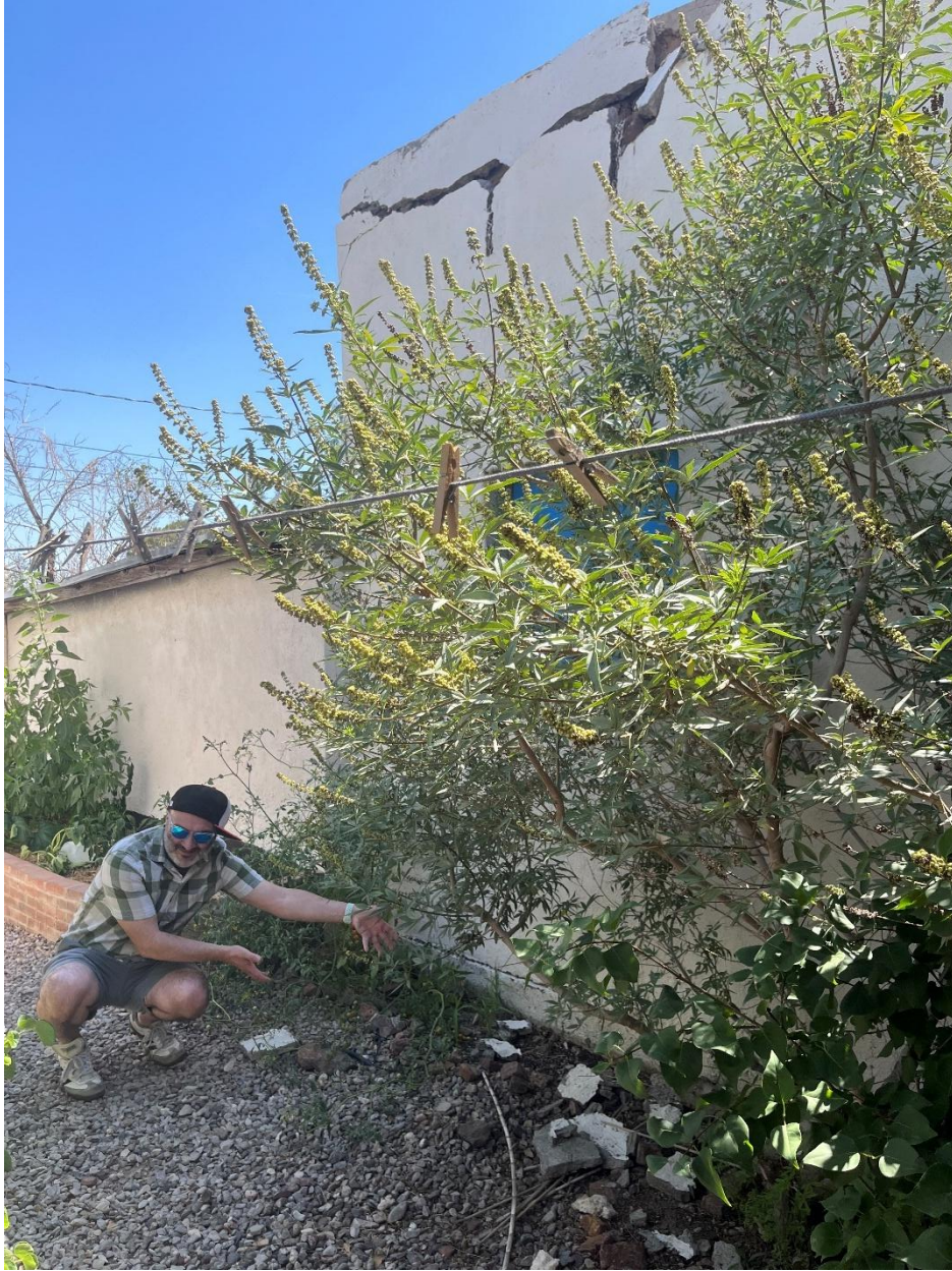
Figure 14: Chunks of plaster that have fallen from the rear of property at 414 E. May into the property at 422 E. May. Photo taken July 9, 2025.
