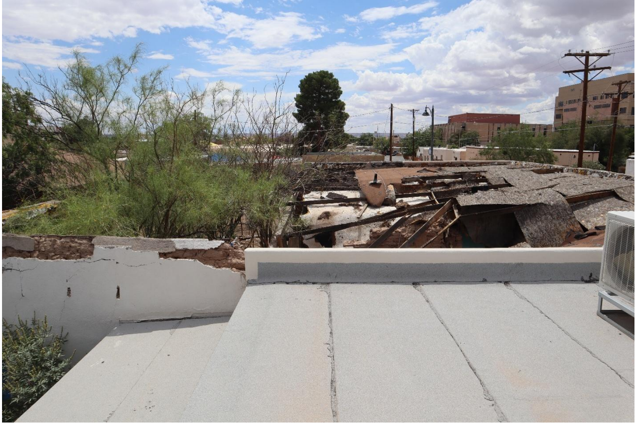
Figure 11: Photo of collapsed roof at 414 E. May from the roof on 422 E. May. Photo taken July 1, 2025.
