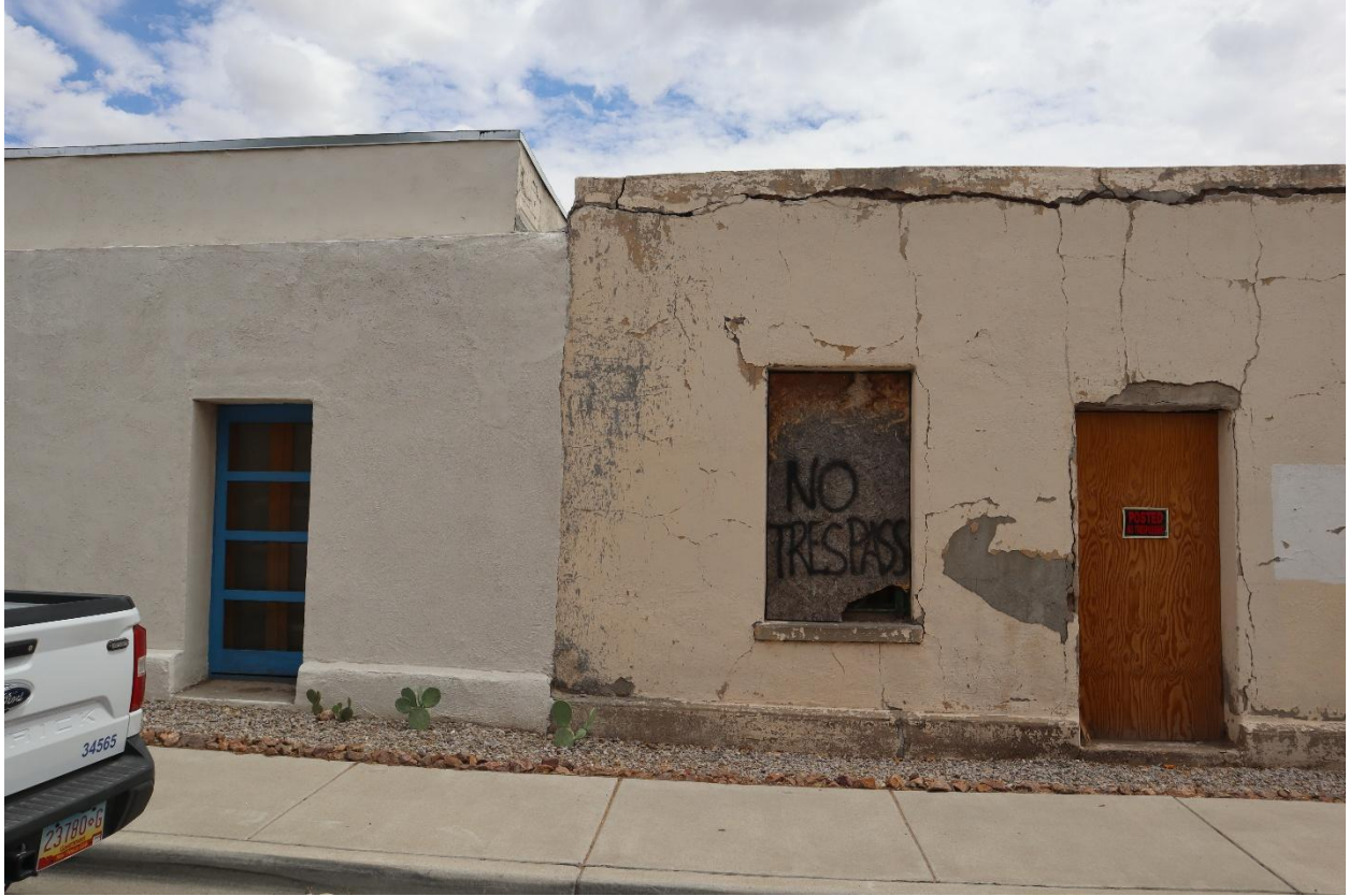
Figure 2: Party wall between 422 E. May and 414 E. May. Photo taken July 1, 2025.
